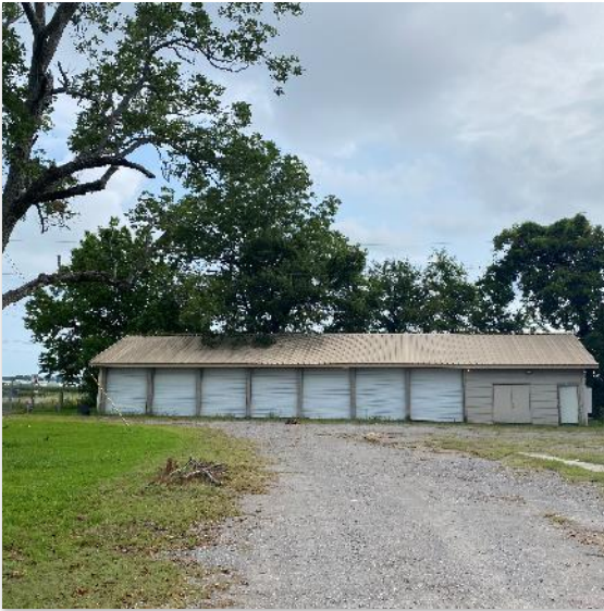
Building 3, Viewed Northeasterly
