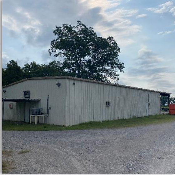
Building 2, Viewed Easterly
