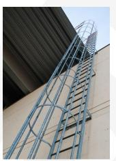
Fixed ladders are permanently mounted to a structure
